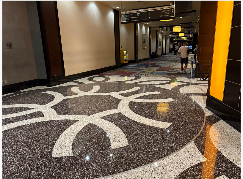
ZINC DIVIDER strips form curved patterns in the epoxy terrazzo installation by Corradini Corp.
