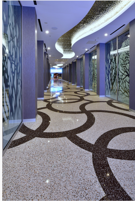
MOTHER-OF-PEARL, mirror and marble chips catch the light in a dazzling terrazzo installation that reflects the city's signature glamour.
