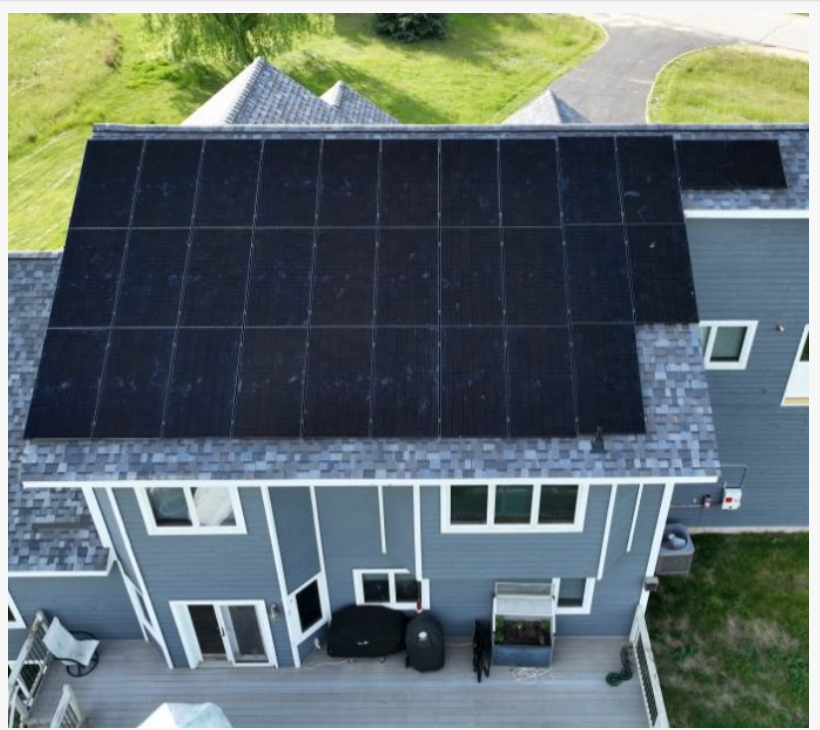
Wolf River Electric - Fully Paneled Roof
