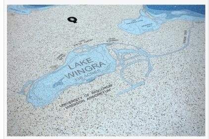
WATERJET TECHNOLOGY was used to cut precise topographical lines in zinc, ensuring accurate scale.
