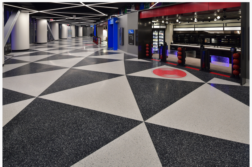
HANDCRAFTED TERRAZZO in the Intuit Dome was poured in place.
