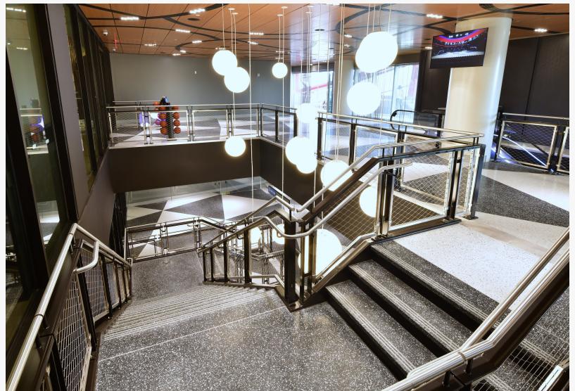
STAIRCASES IN PRECAST terrazzo connect all levels of the sports and entertainment arena.
