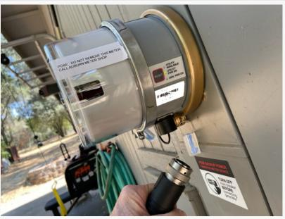
The generator cable simply plugs into the collar. The BPTM does the rest.
