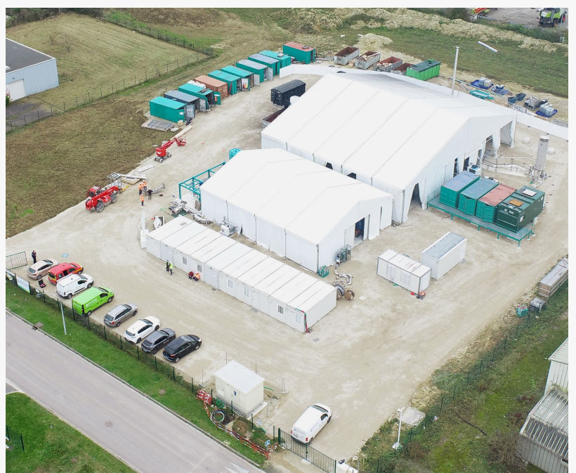
Haffner Energy's center of hydrogen production, testing and training in Vitry-Marolles industrial zone.
