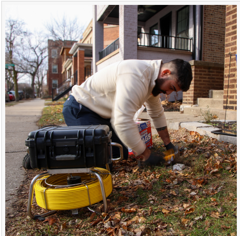
A J. Blanton Plumbing technician assisting a Chicago homeowner with plumbing maintenance, preventing costly post-winter repairs by addressing clogged drains and performing a sewer cleanout.
