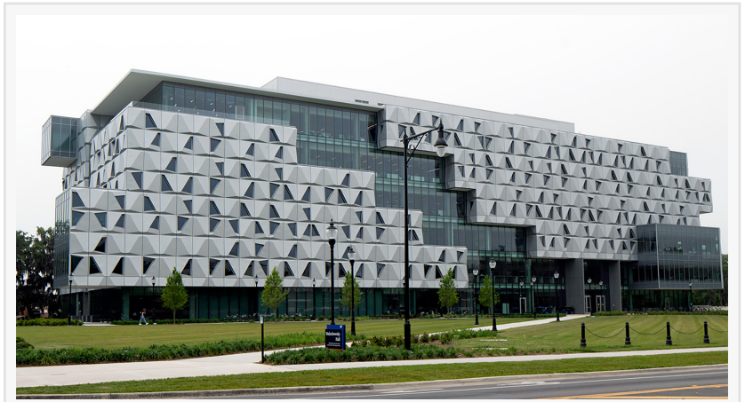
Malachowsky Hall North Elevation (Main Elevation) Facing Reitz Union Another view of the north (main) elevation of Malachowsky Hall, where N-RG Cladding LLC’s advanced facade design integrates post-painted aluminum panels and architectural glass. Facing t
