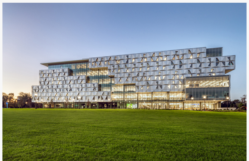
Malachowsky Hall North Elevation (Main Elevation) Facing Reitz Union The north (main) elevation of Malachowsky Hall for Data Science & Information Technology at the University of Florida, featuring N-RG Cladding LLC's prefabricated exterior system. This v
