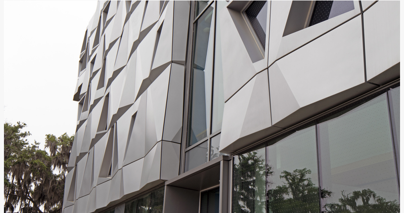
Malachowsky Hall East Elevation Entry with Volumetric Panel Geometry The east entry of Malachowsky Hall at the University of Florida, emphasizing N-RG Cladding LLC's volumetric panel geometry. Distinct angles, modular panels, and careful engineering highl
