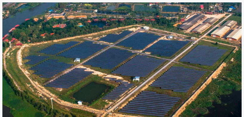
Recent Solar Project
