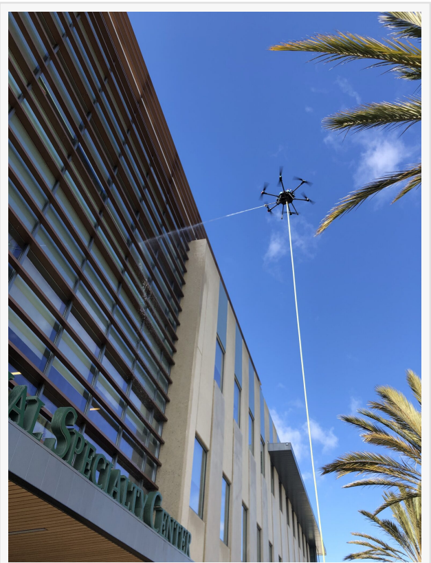
SprayTech’s FAA-certified drone cleaning the exterior of the Specialty Center at Torrance Memorial Medical Center (TMMC), ensuring safe, efficient, and cost-effective maintenance.
