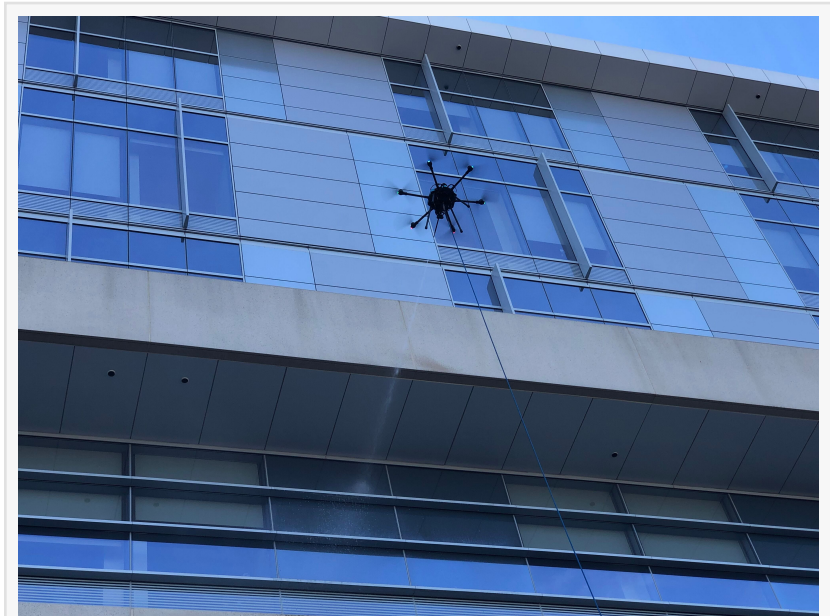
SprayTech's FAA-certified drone cleaning the exterior of Lundquist Tower at Torrance Memorial Medical Center (TMMC), providing a safer, cost-effective alternative to traditional maintenance.
