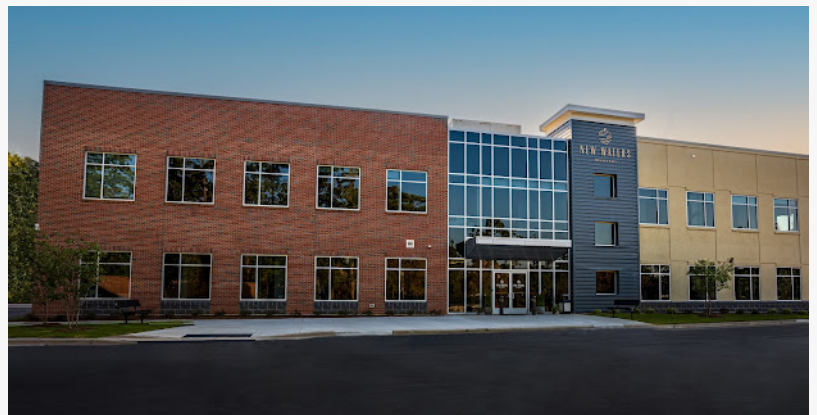
New Waters Recovery Building
