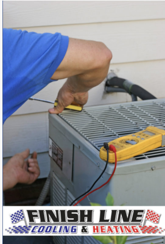
AC Repair - Finish Line Cooling & Heating
