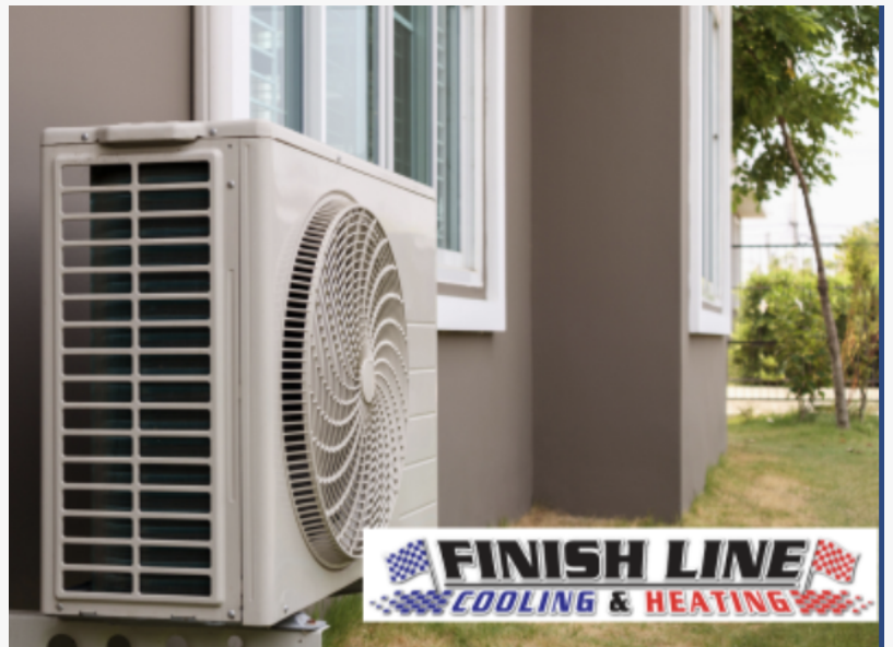
Air Conditioner Installation - Finish Line Cooling & Heating
