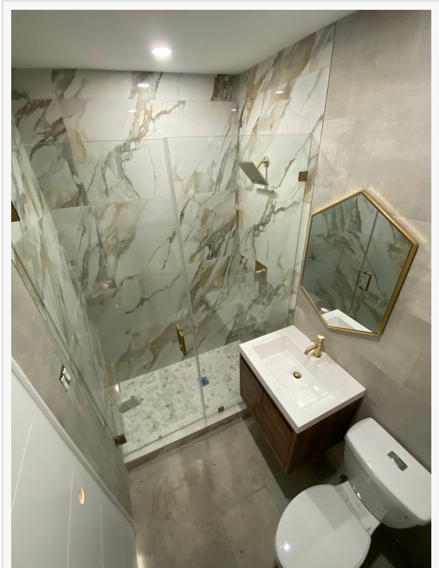
Lumina Construction, Expert Bathroom Renovations in NYC
