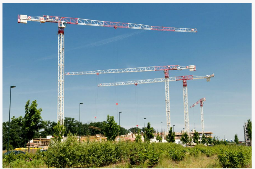
Tower Crane Rental 1
