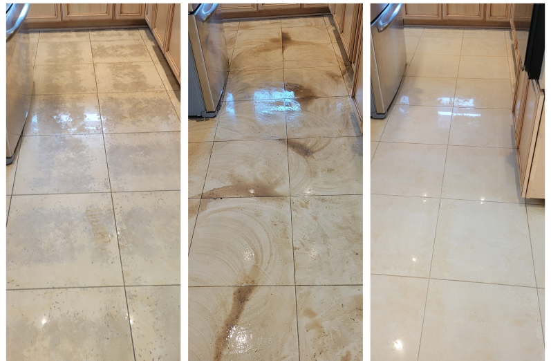
3 panel photo of tile and grout cleaning: dirty, scrubbed, cleaned
