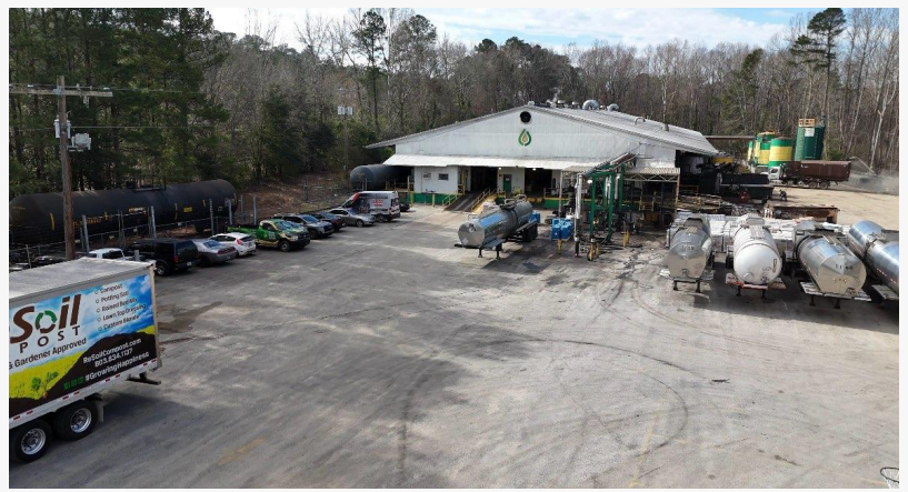
Green Energy Biofuel's grease-processing facility in Warrenton, South Carolina.
