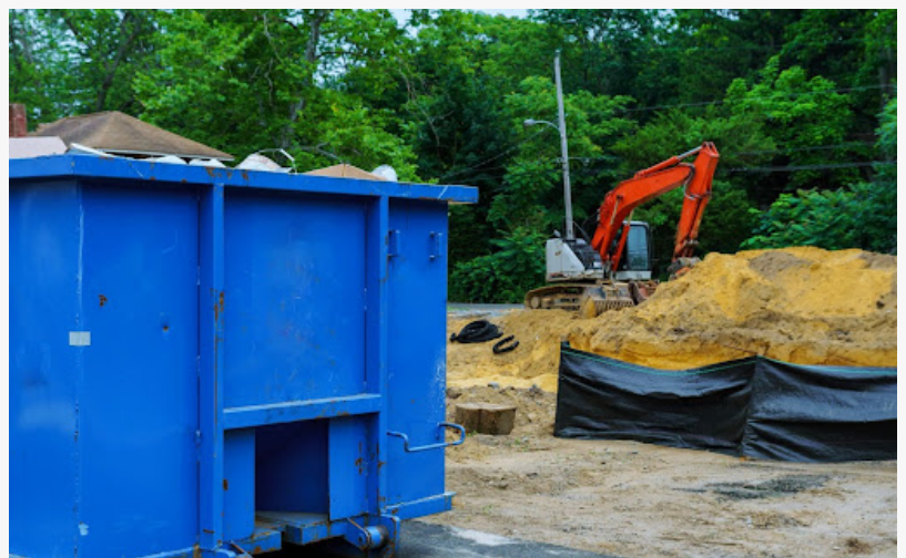
A blue commercial dumpster on a construction site.
