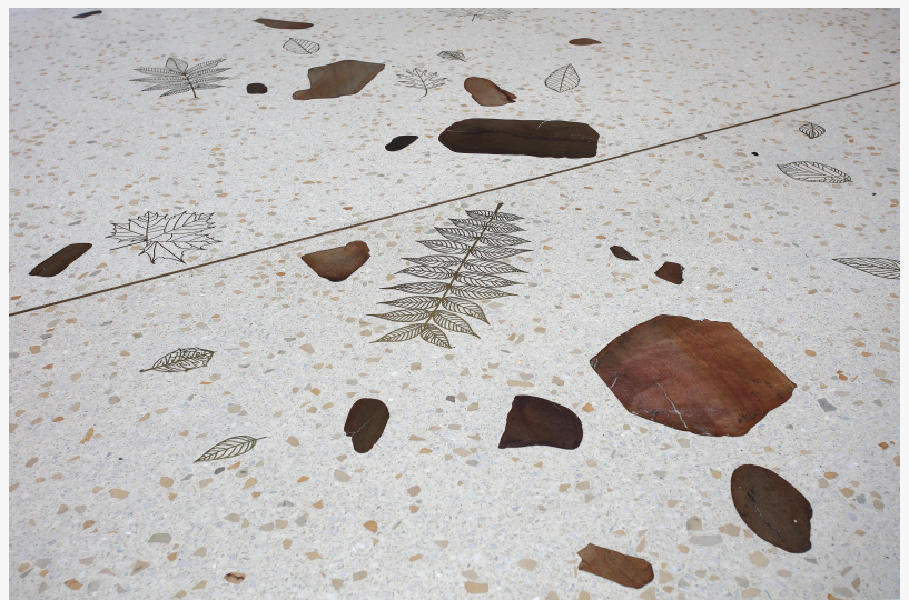
HAND-CUT river stones and over 800 waterjet-cut brass leaves are embedded in the terrazzo floor at the Missouri Botanical Garden's new visitor center.
