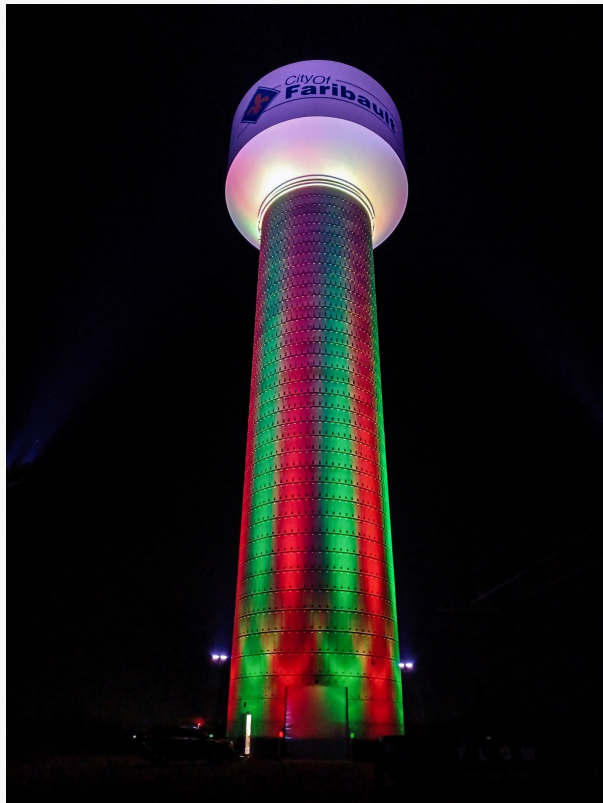
View of Elevated Water Tank in Faribault, MN
