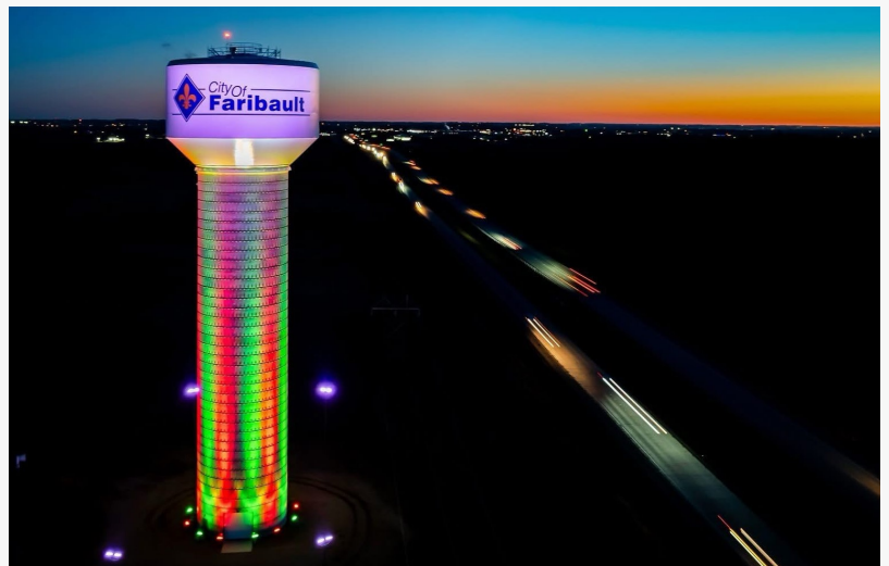
Elevated Water Tank in Faribault, MN
