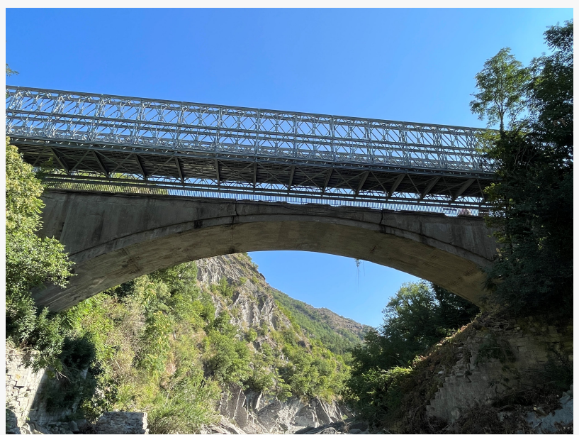
Acrow Bridge - Santerno Toscana Italy
