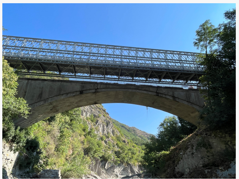
Acrow Bridge - Santerno Toscana Italy
