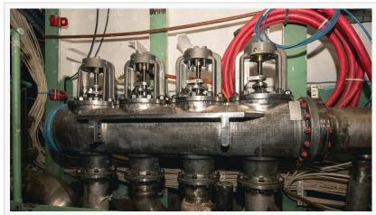
DM3D manufactured valve manifold assembly, a specialized assembly that allows distribution of a single source of fluid to multiple points on the ship, is installed in a pump room on Gerald R. Ford-class aircraft carrier Enterprise (CVN 80)
