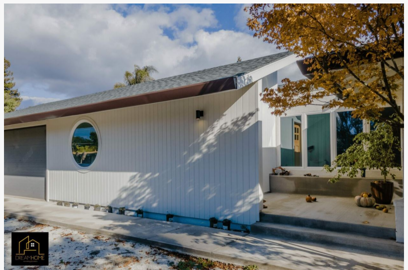
Home Addition Expansion in the Bay Area, California
