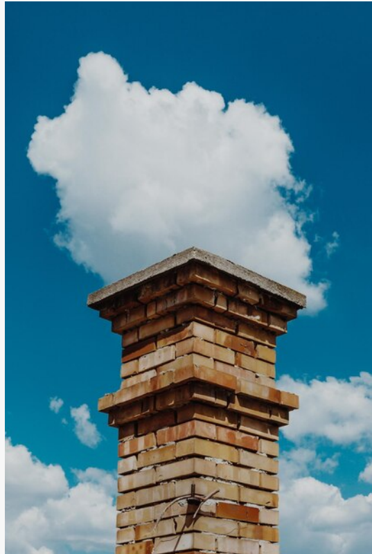
chimney repair service
