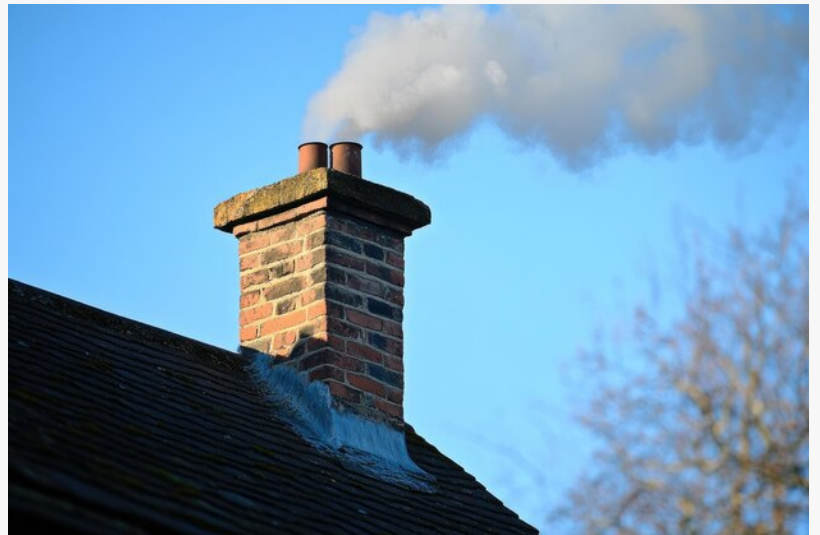
chimney and masonry services
