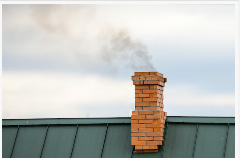
chimney leak repair
