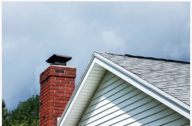
best chimney repair near me
