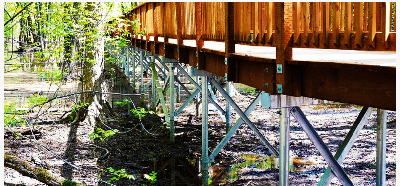
Boardwalk Constructed With Pressure Treated Lumber
