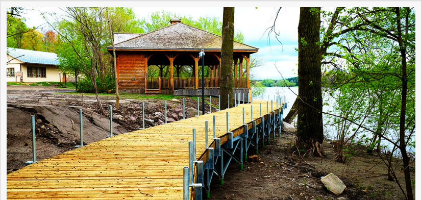
Eco Friendly Helical Pier Boardwalk
