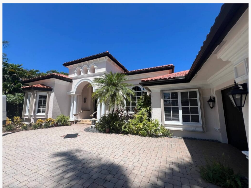
Exterior Painting Solutions Painting
