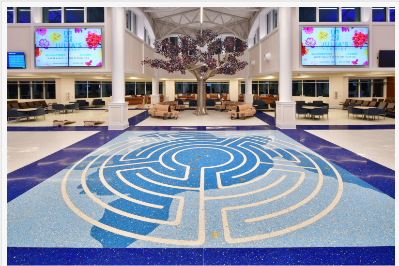
THE AWARD-WINNING TERRAZZO installation welcomes travelers to Wilmington International Airport with a loggerhead labyrinth with seashell aggregates. (David Laudadio, courtesy of David Allen Company)
