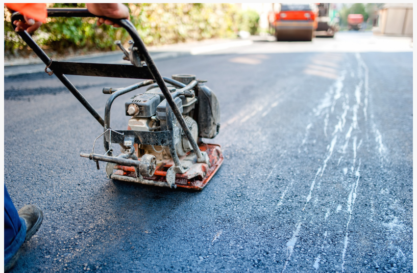
Oscar's Asphalt & Sealcoating in Essex County, NJ
