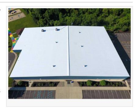
Acrylic coatings are composed of advanced polymers engineered to provide both strength and flexibility. These coatings form a seamless elastomeric membrane that adheres fully to roof
