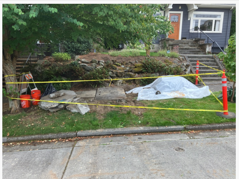
Residential home undergoing sewer repair
