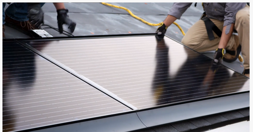
Simmitri Inc. Solar Installation
