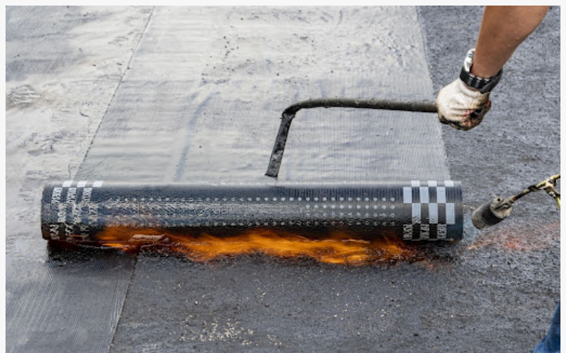
Torch down specialty roofing used to waterproof a multi-storey residential building.
