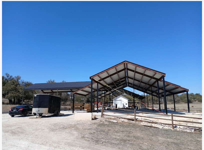
Steel Framed Barn Under Construction
