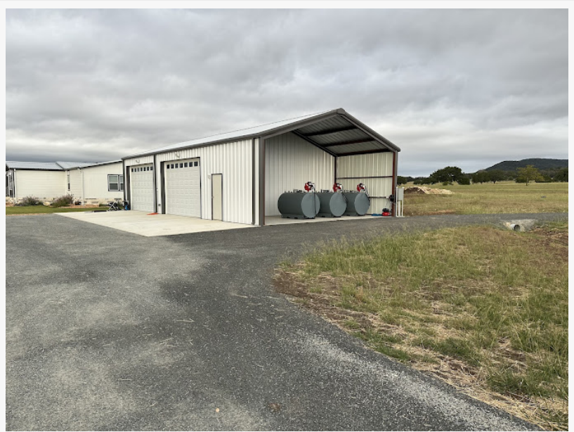
Custom Steel Garage with Fuel Tanks
