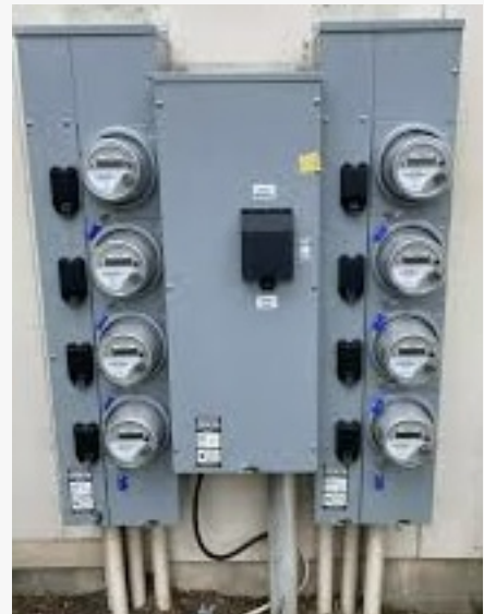
Exterior Multiple Meter Panel
