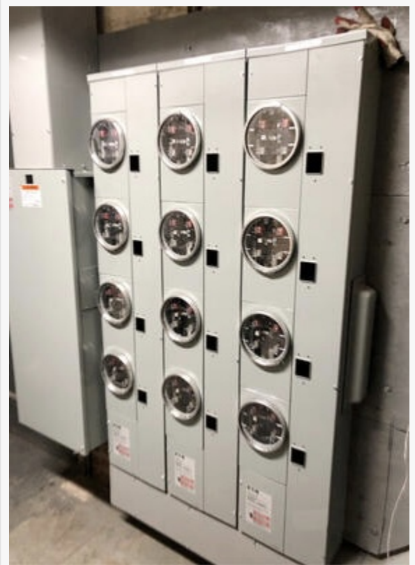
New replacement electrical panel with meters
