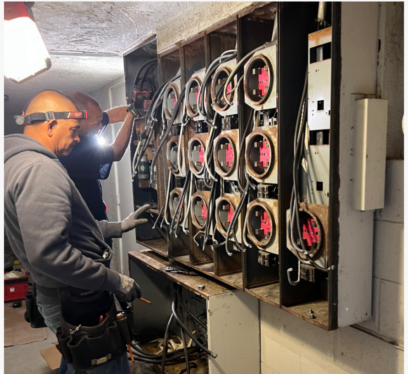
Replacing a multiple meter panel
