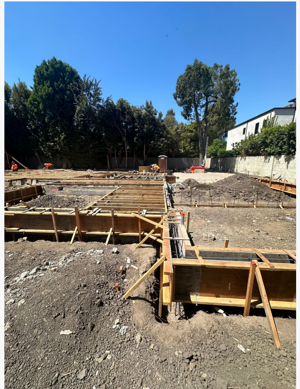
The S&P Concrete Construction crew prepares a residential foundation for a new ADU in Orange County.
