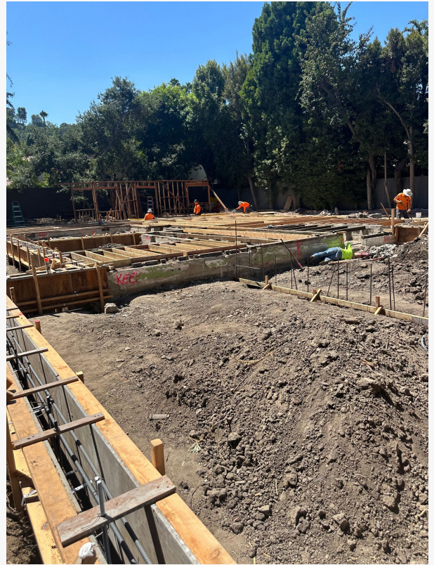
The S&P Concrete Construction crew frames a multi-section ADU foundation during an active build in Los Angeles County.
