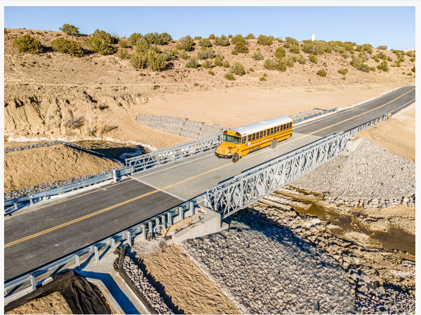
Acrow Bridge in Cibola County, New Mexico
