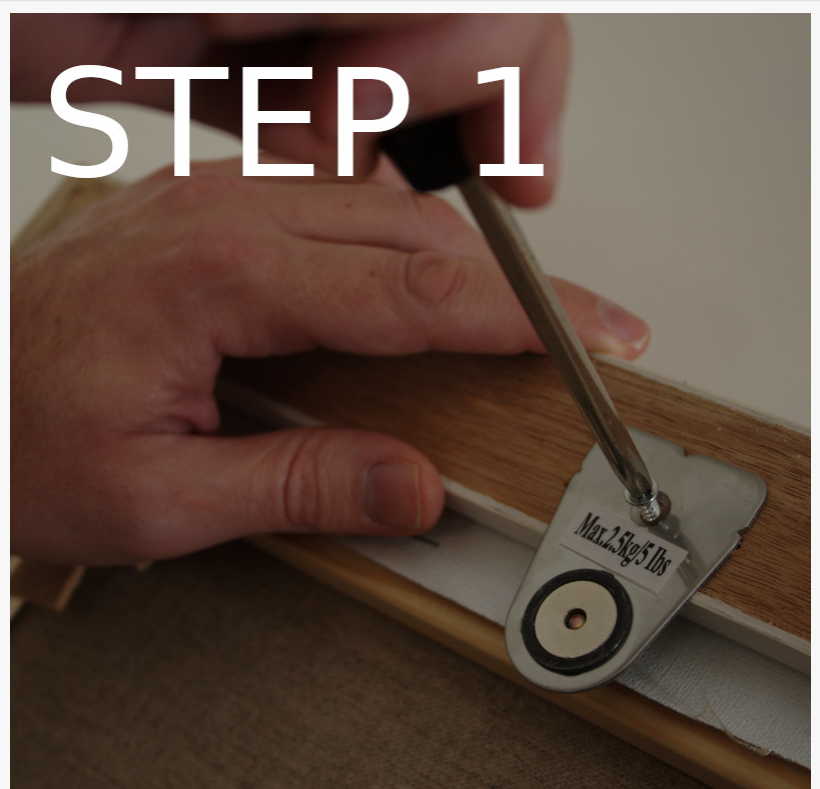
Step 1 fix the two magnets at the top and bottom of the back of frame
