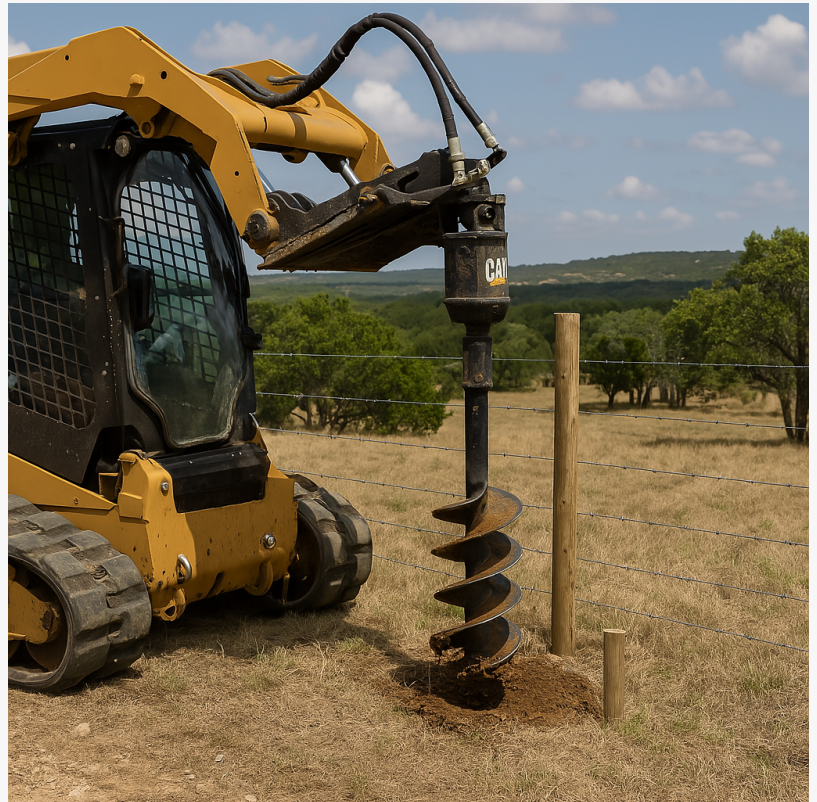
Fredericksburg Texas auger fence installation installer
