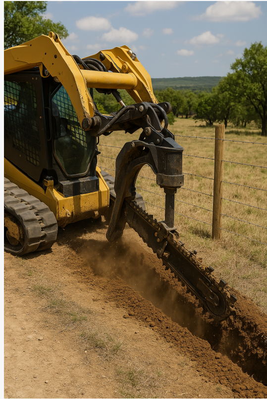
Fredericksburg texas trenching trencher service
