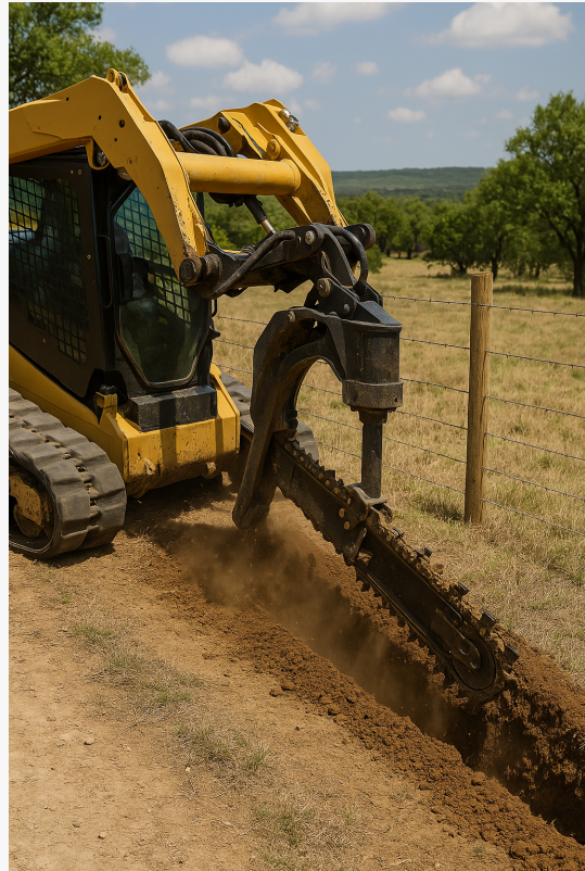
Fredericksburg texas trenching trencher service
