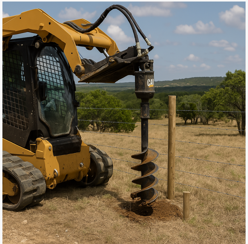
Fredericksburg Texas auger fence installation installer
