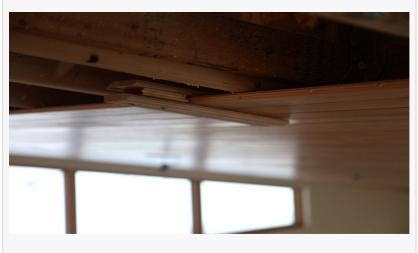
boards in place prior to nailing, ensuring proper alignment and reducing the risk of mistakes.
