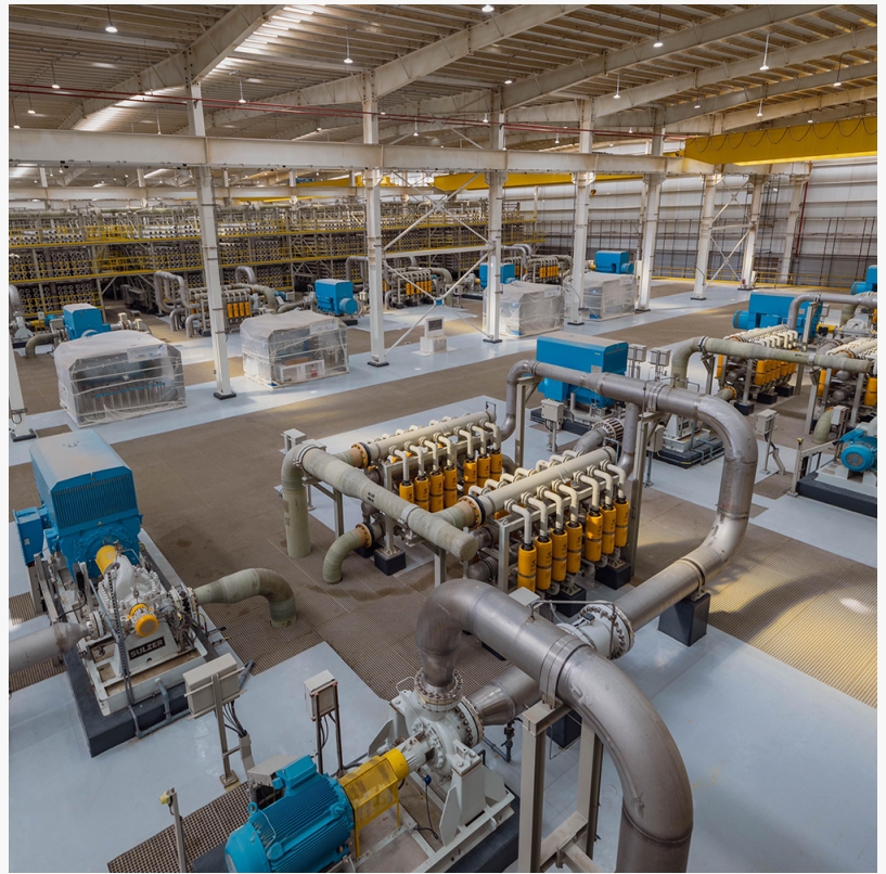
A glimpse of the cutting-edge reverse osmosis system at Shuaiba-5, showcasing advanced membranes and energy-efficient pumps.
