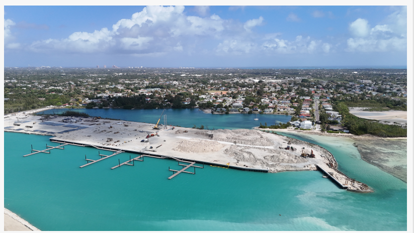
April 2025 Construction Progress
