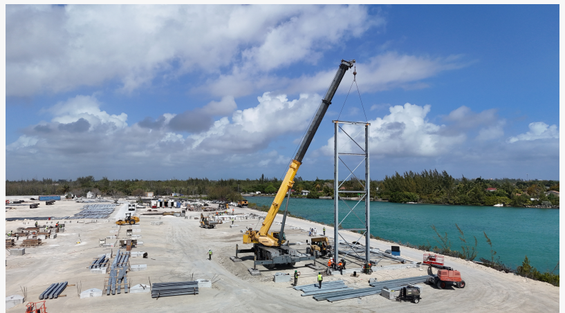
Steel Construction Erection
