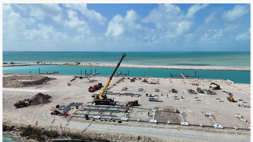
Dry Storage Construction Begins At Blue Water Cay
