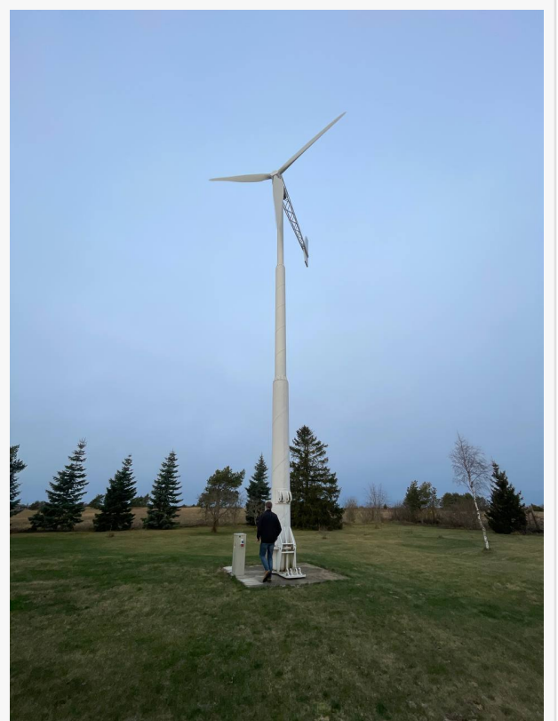
Freen-H15 small wind turbine
