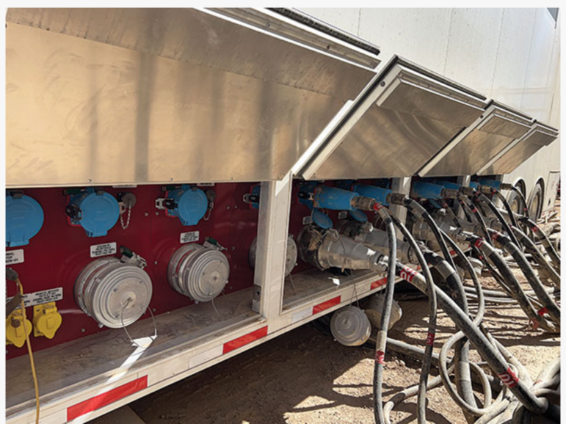
MELTRIC DS200 Oil Drilling Power Distribution
