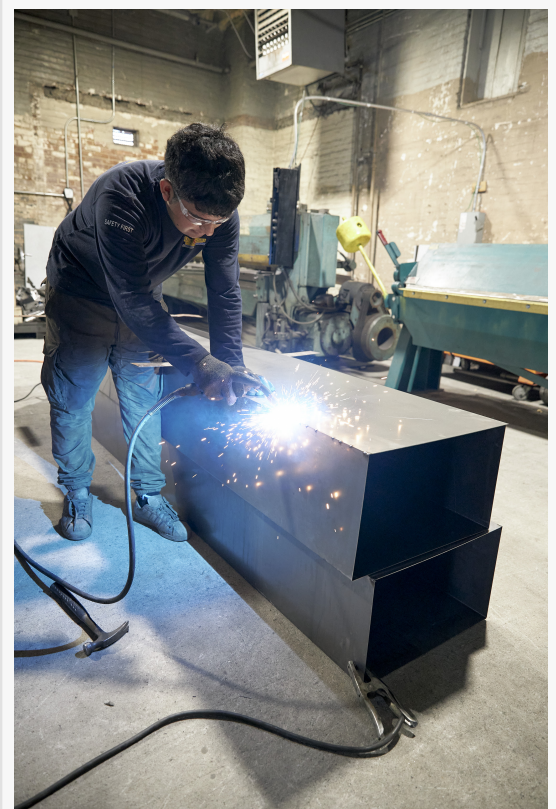
Done Right fabrication team welding a NFPA 96 code-compliant exhaust systems.
