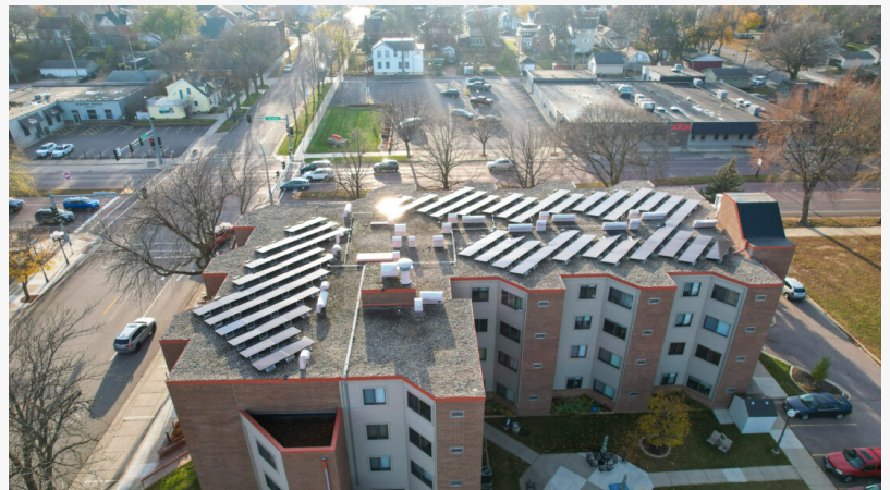
New Ulm Solar Public Housing Installation
