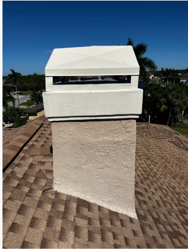
Chimney Cap Installation Florida -
