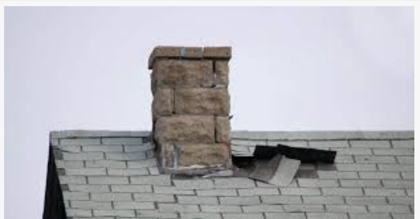
leaking chimney repair florida
