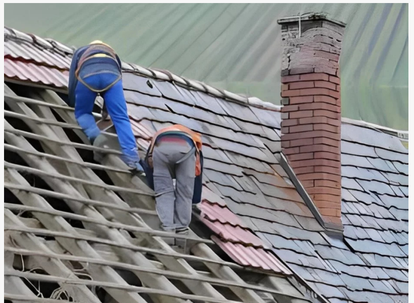
chimney leak repair Florida
