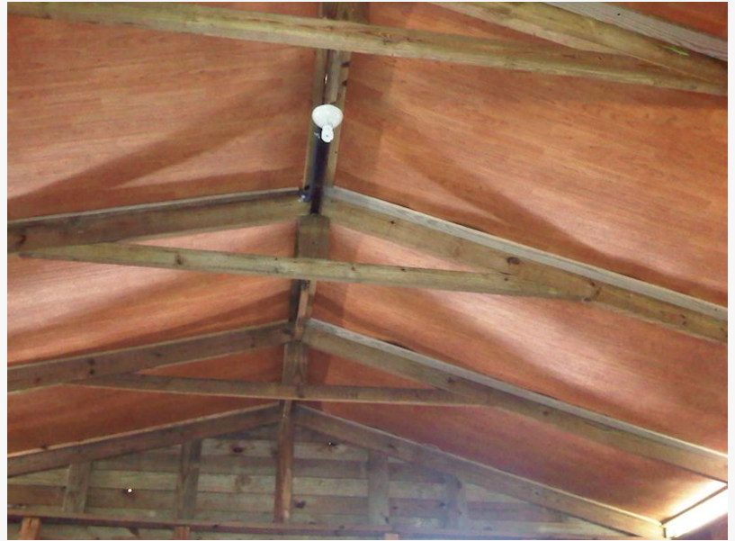
Rustic Prodex Total Insulation roll in ceiling/roof
