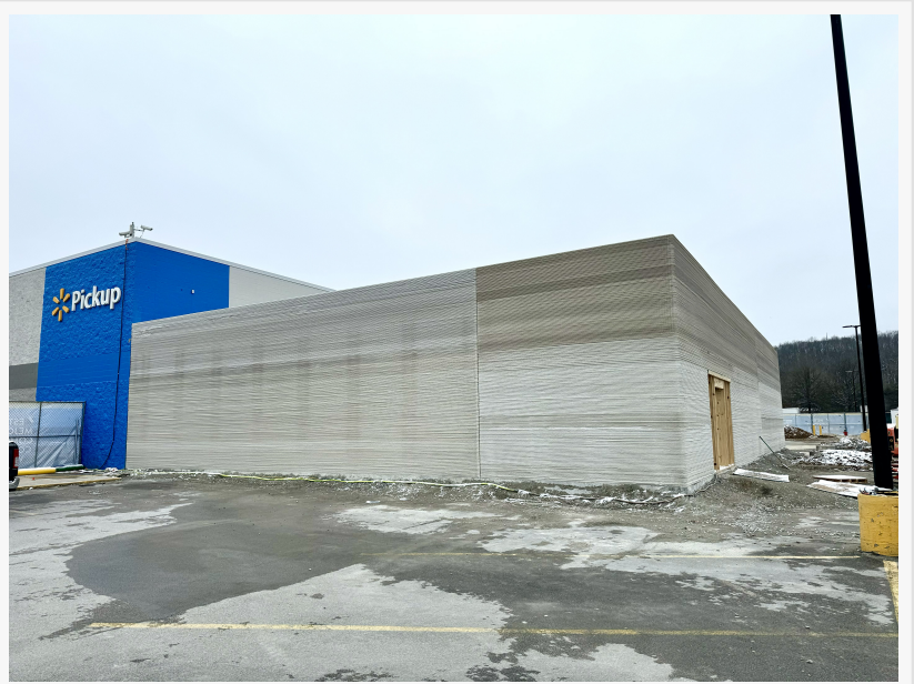
Finished Walmart extension
