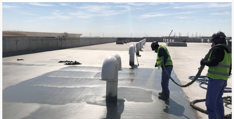
Roof coating with VIPShield system
