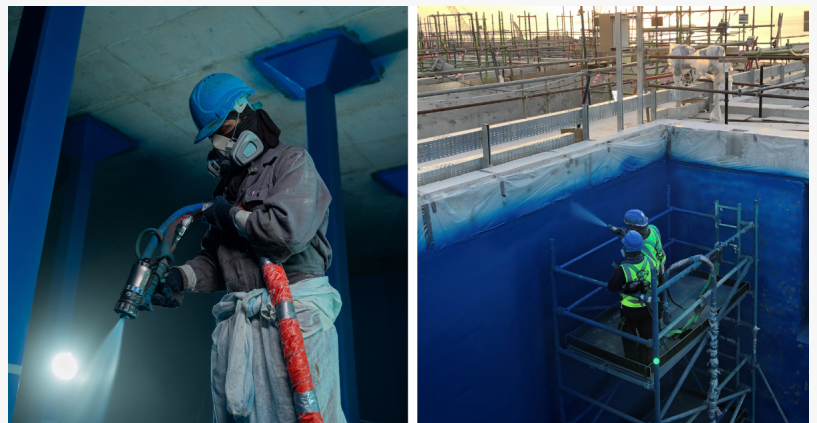
Potable Water Tank Coating with Liquishield
